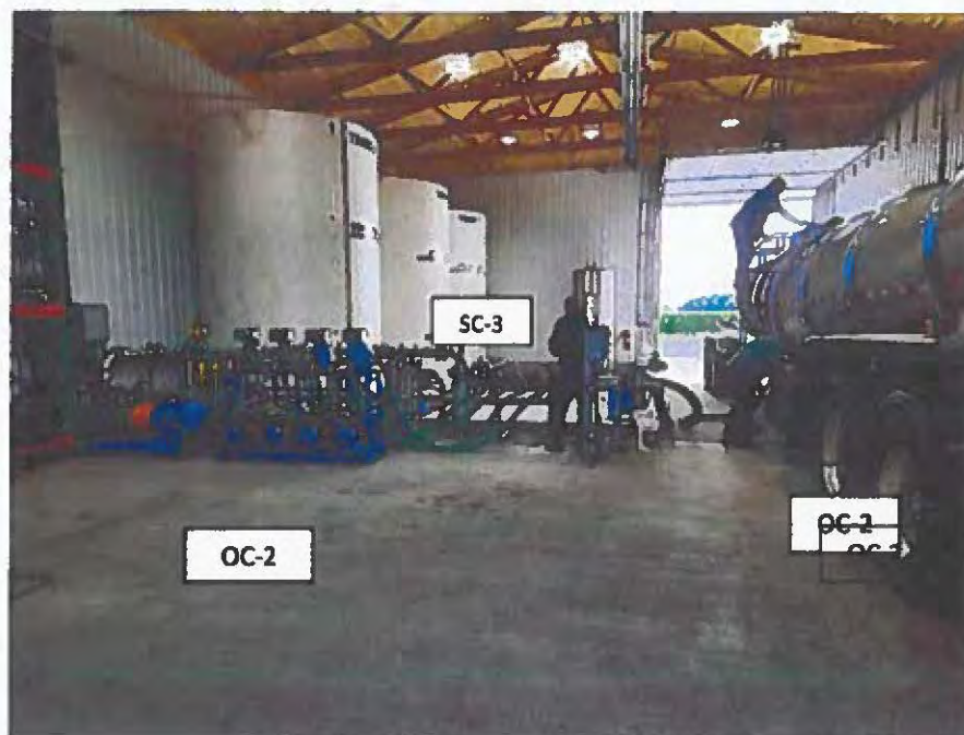
Figure 3- Inside View of OC-2 and SC-3
