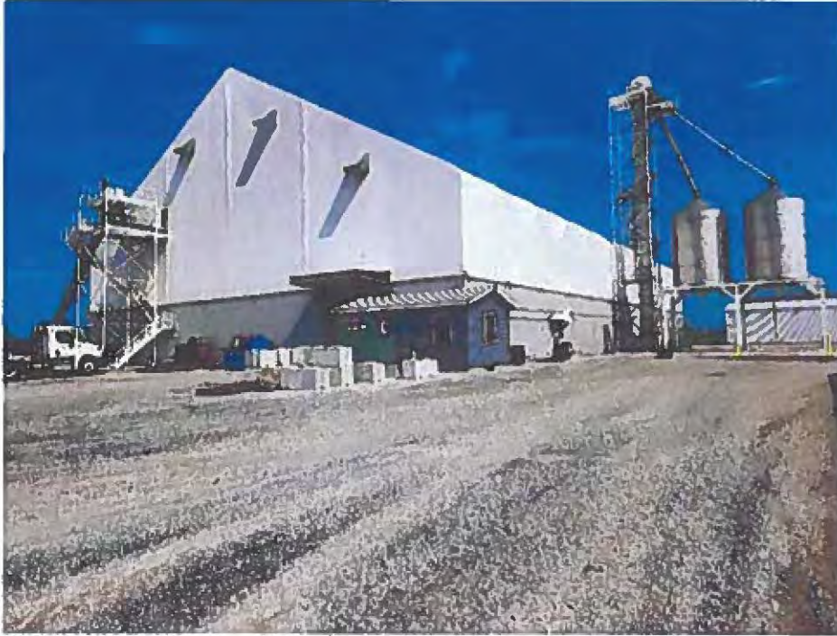
Cisne Dry Fertilizer Storage and Operational Building
