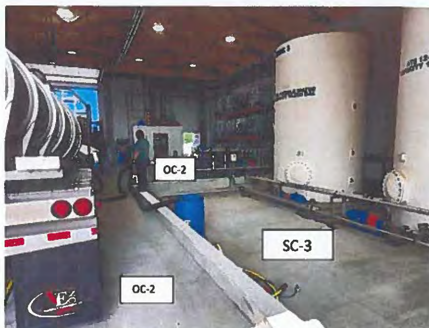
Figure 2 - Inside view of OC-2 and SC-3
